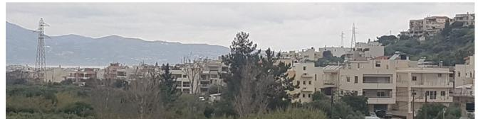
Fig. 4. View of three lattice towers of an out of service 66 kV OTL which used to span over residential areas in Heraklion. All conductors and the overhead ground wire have been removed.
