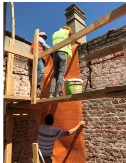
Fig. 8. The reinforcement of brick walls
