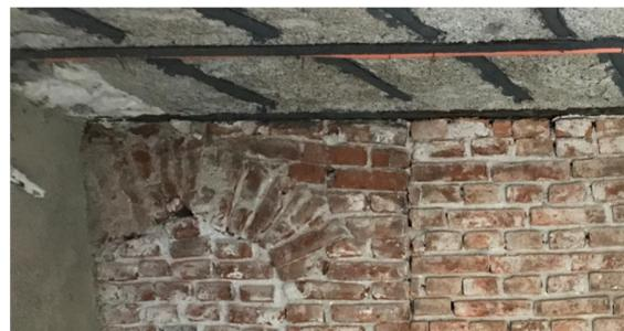
Fig. 13. The reinforcement of the R.C slab in the entrance of the building
