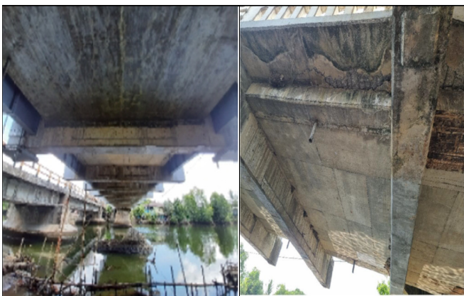
Fig. 5. Visual condition of the Pute Bridge-river deck slab.
